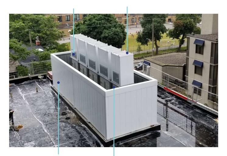
PMA 'AcoustaMod' Acoustic RT Barrier (Structure Mounted) Attentuates Intake Noise
