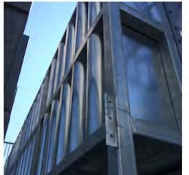
As previously reported, cranes were seen lifting equipment on to the roof of 252 Sackville Street in late June. The parts were assembled the week prior to Canada Day, and the silencers seem to be doing their job since even under high heat and humid conditions, the noise from the Energy Centre has been largely reduced. It is still audible outdoors when running at full speed, but the level blends into background noise such as traffic from TCHC sent us this photo of part of the silencer of
